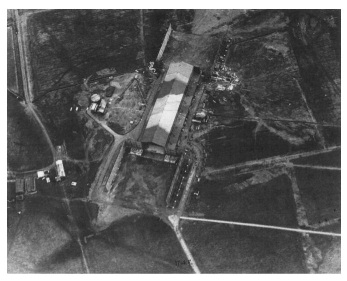
*View of RNAS Llangefni taken from an airship in 1917. Note the windshields at the ends of the shed and the gas plant to the left (Courtesy of Anglesey Archives).*
