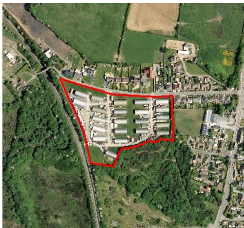
Above Next Perspectives aerial photo mapping, and below Google street view 2011.
