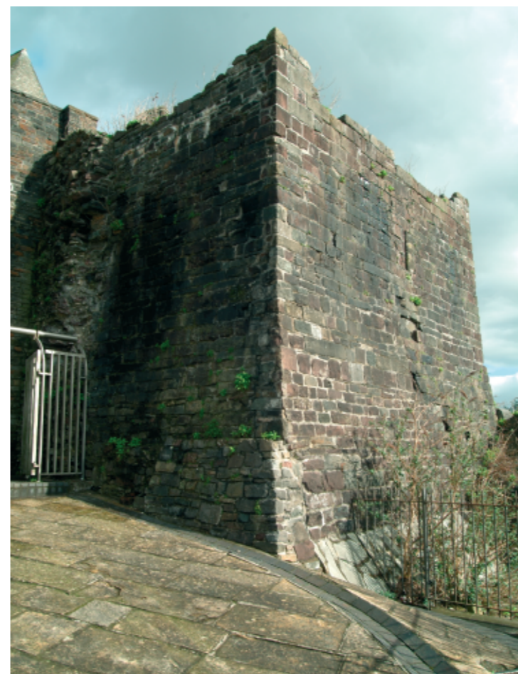
Y Tŵr Sgwâr o'r de-orllewin The Square Tower from the southwest
