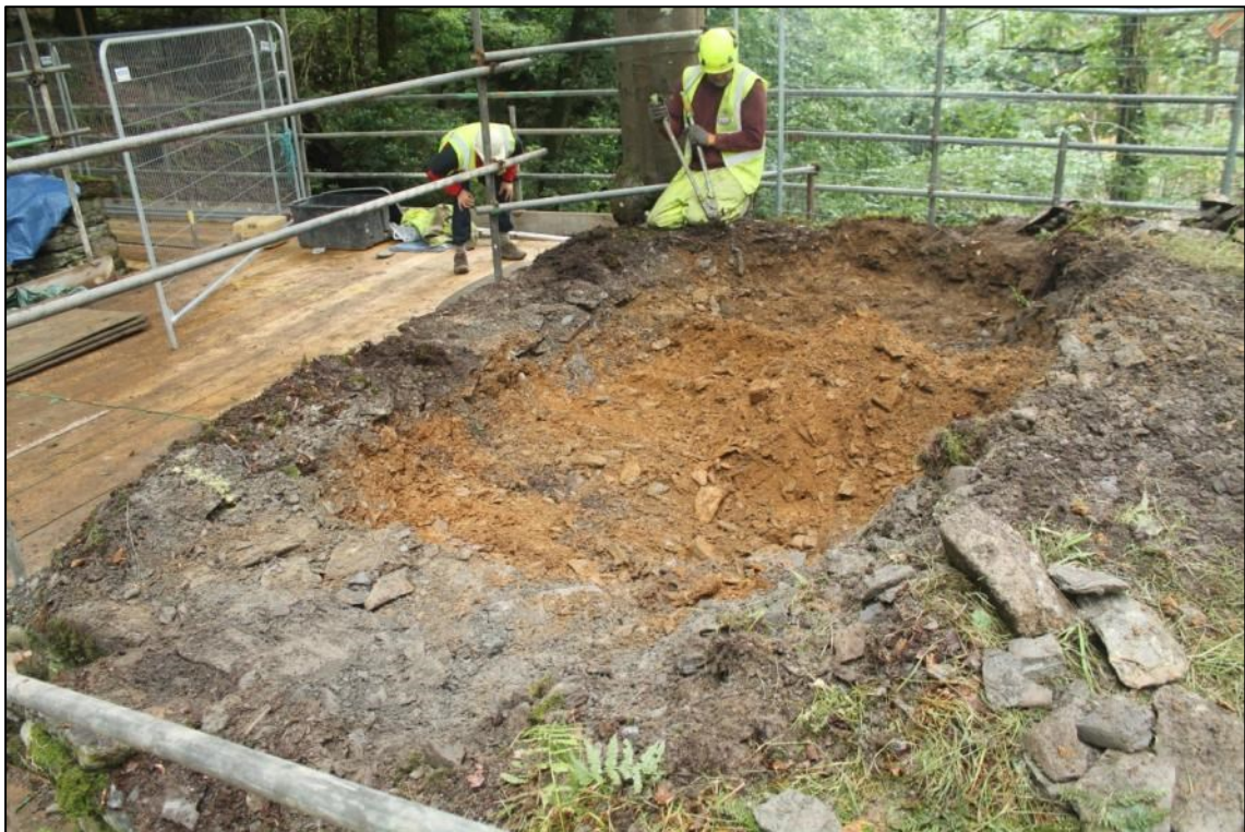
Photo 14: The orange subsoil infill (203) revealed in the north-western abutment (DAT Photo 110511_0034).
