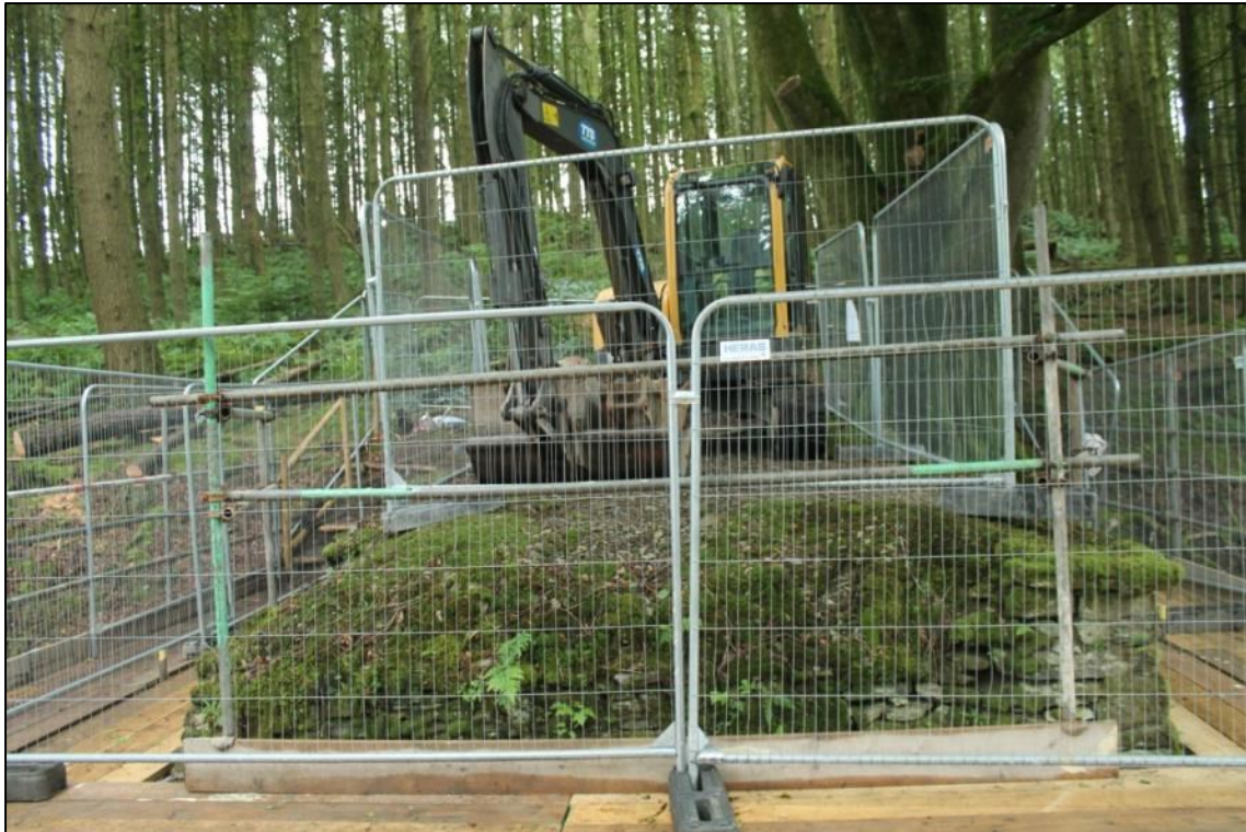
Photo 2: The south-eastern bridge abutment prior to works (DAT Photo 110511_0001).
