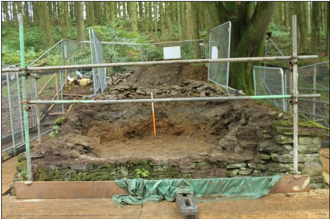
Photo 11: The section of the abutment infill and the reduced walls at the end of the excavations of the south-eastern abutment (DAT Photo 110511_0024).
