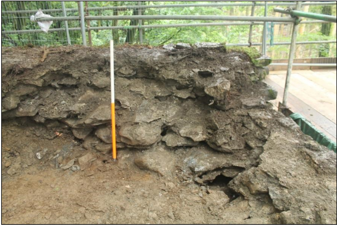
Photo 8: The partially dismantled internal face of the southern wall of the south-eastern abutment (DAT Photo 110511_0026)
