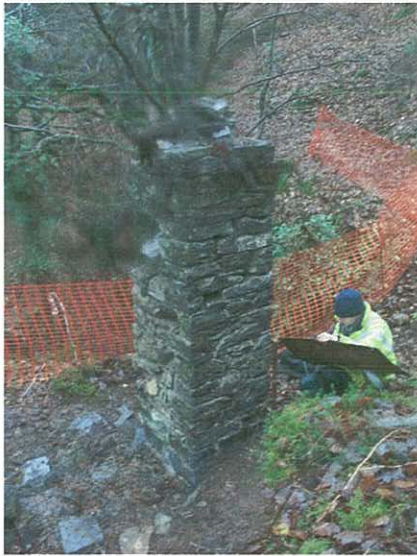
Illustration 7. Southeast pier from the west. 14 November 2002.
