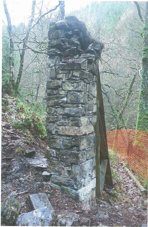
Illustration 4. Northwest pier from the southeast. 14 November 2002.
