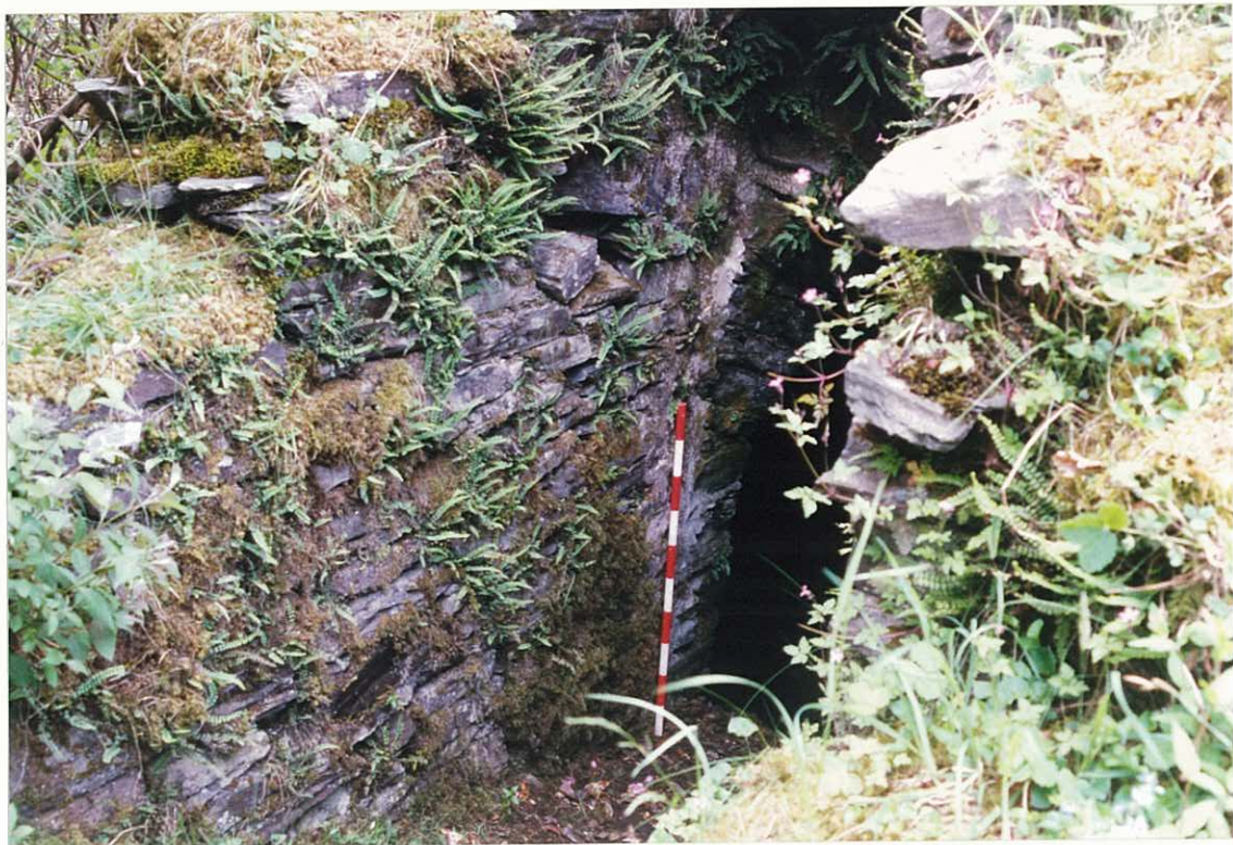
Photo 6. South passageway wall.
