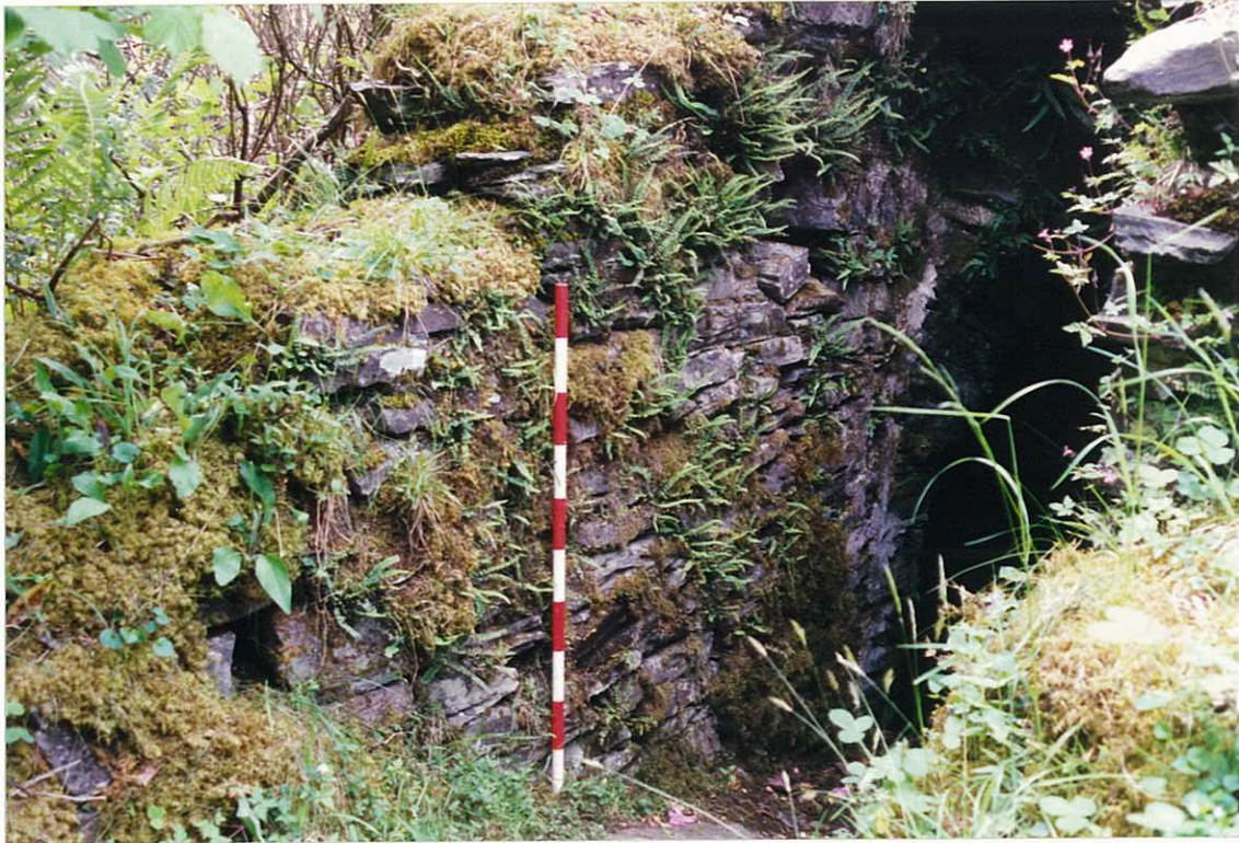
Photo 5. South passageway wall.
