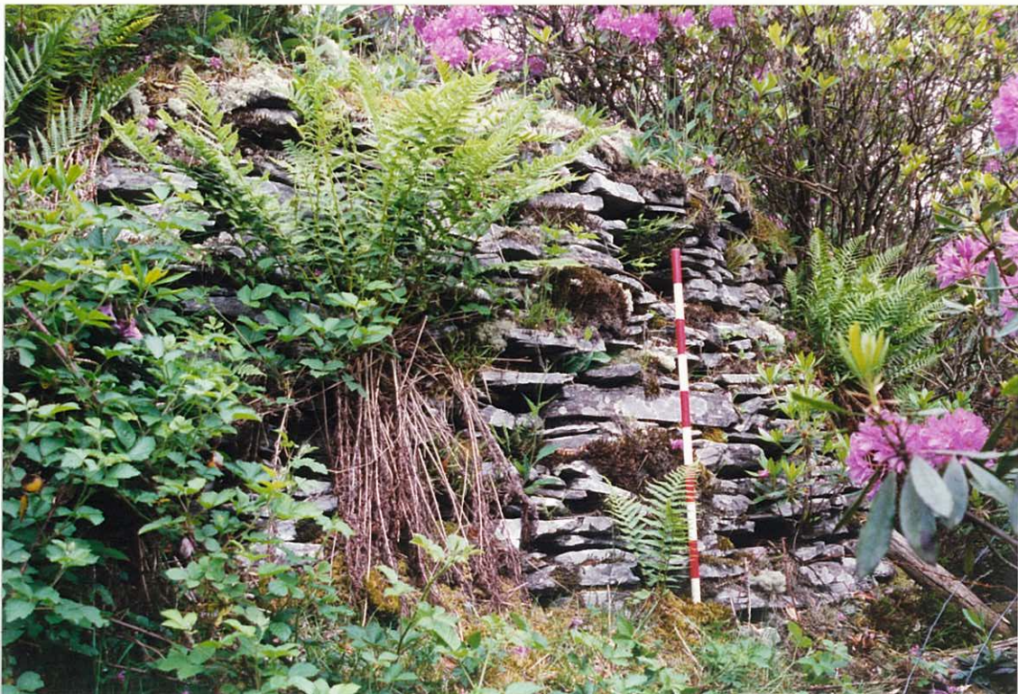
Photo 4. External wall on south side.
