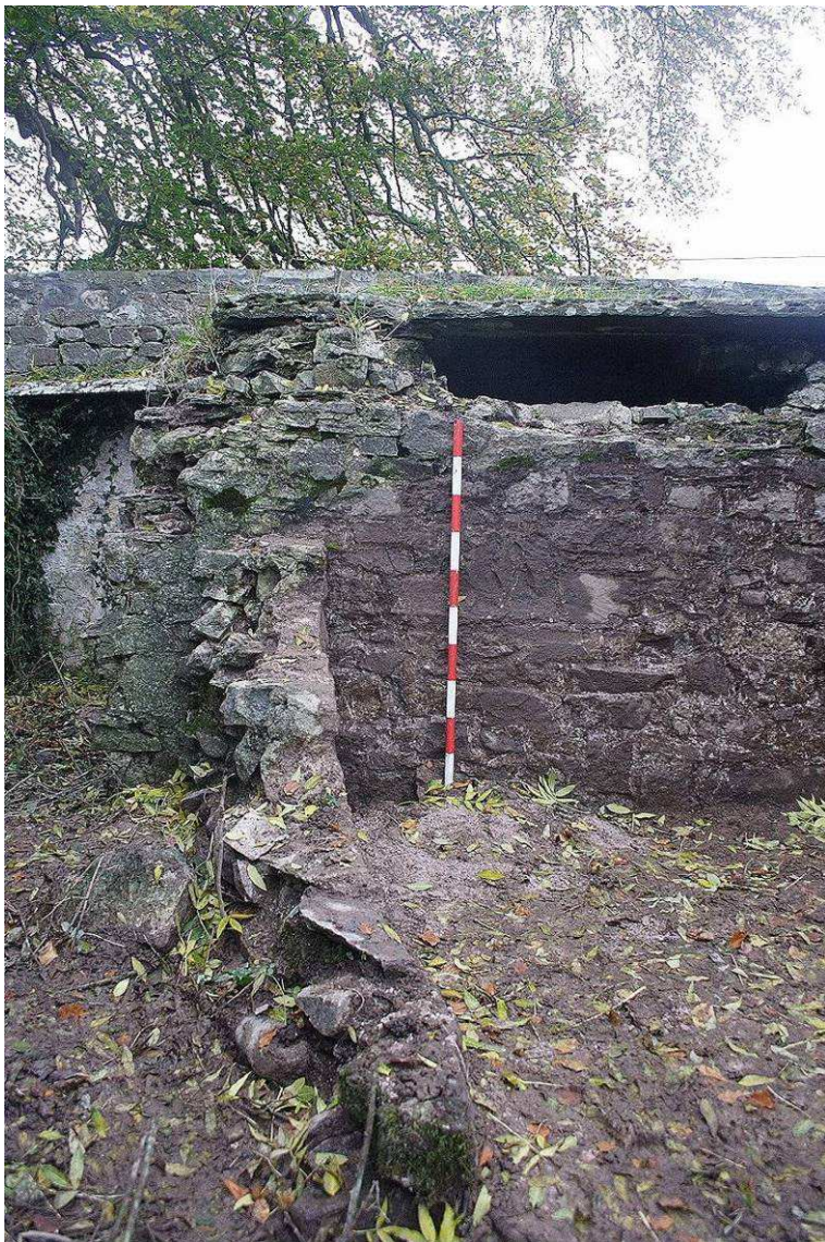
Photo 14: WNW facing shot of Room 2 with attached wall forming an outer enclosure. 1 x 1m scale
