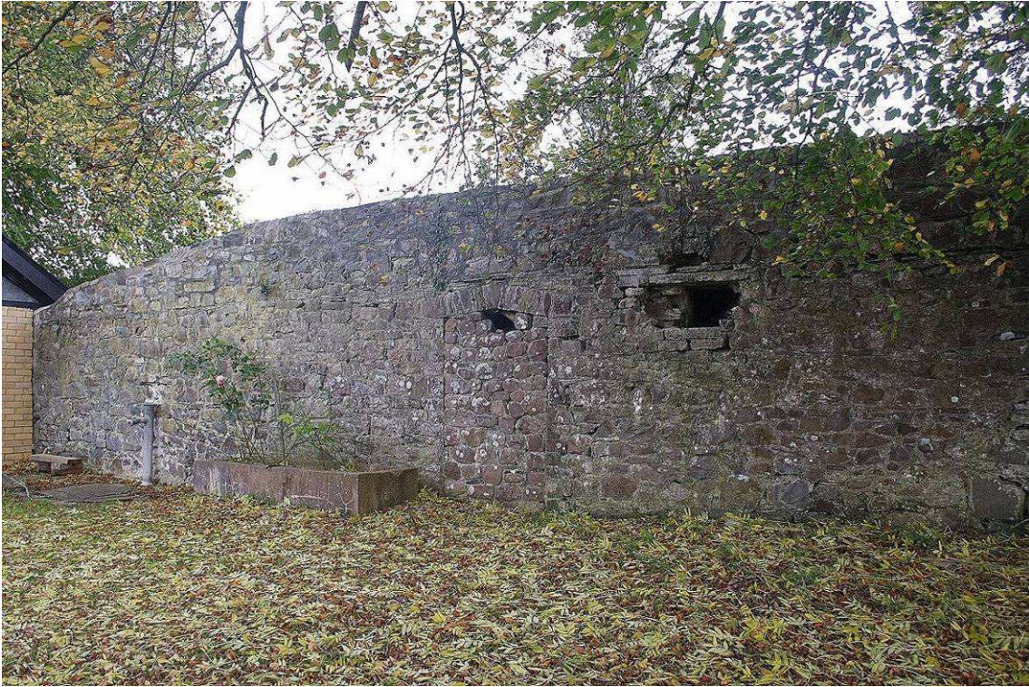
Photo 12: East facing shot of the boundary wall around the former mansion site, showing the blocked doorway entrance to Room 1 and window to Room 2
