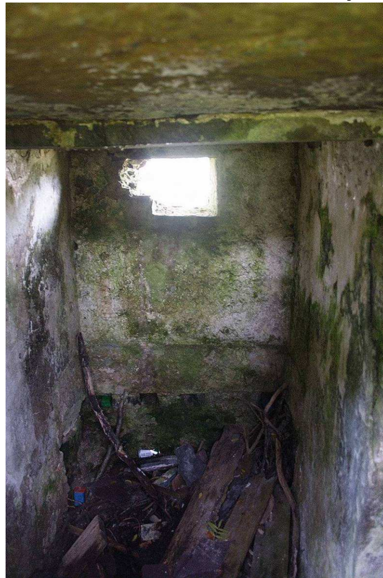
Photo 15: WNW facing shot of the interior of Room 2
