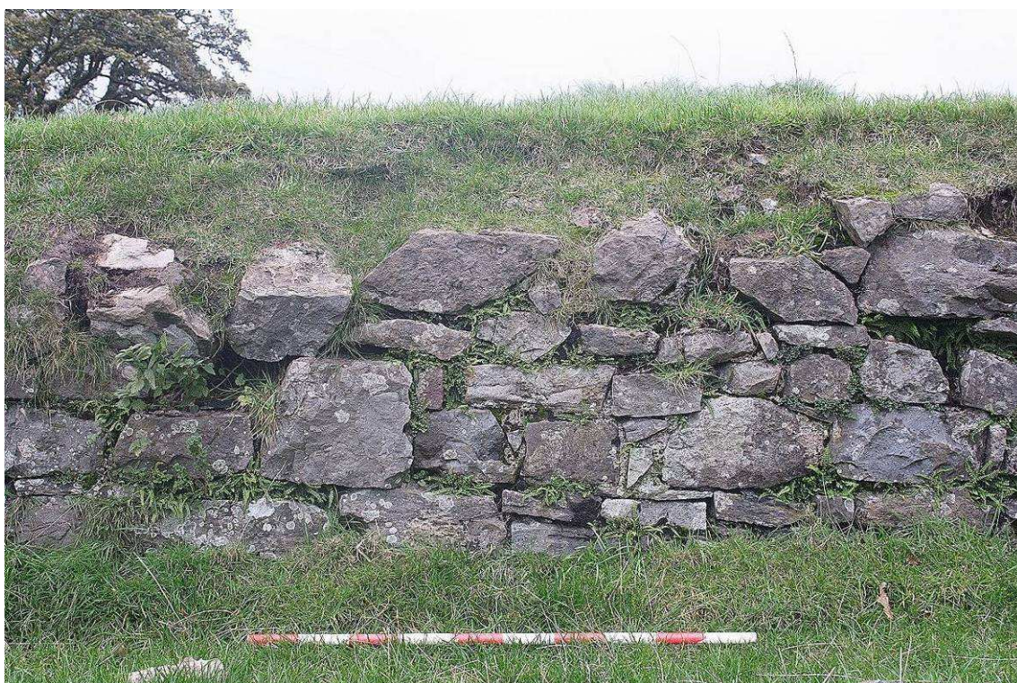
Photo 11: NE facing shot of the boundary/ha ha wall. 1 x 1m scale
