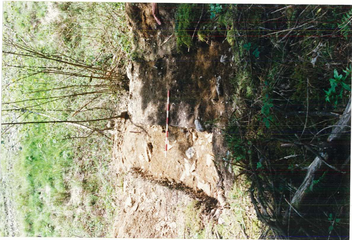
Trench 3 after excavation.
