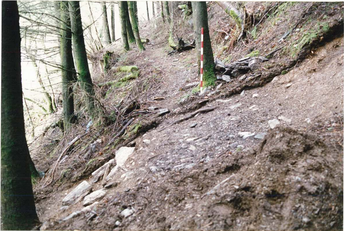
3. Trench 1 after removal of topsoil.
