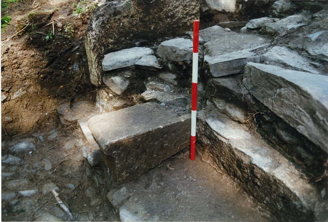
34. Trench 9, detail of step.
